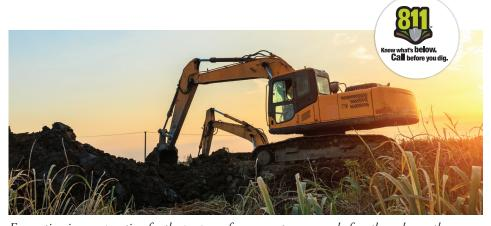
Excavation is any operation for the purpose of movement or removal of earth, rock, or other materials by the use of powered, mechanical or manual means, including digging, augering, boring, backfilling, dredging, plowing-in, trenching, ditching and grading.
