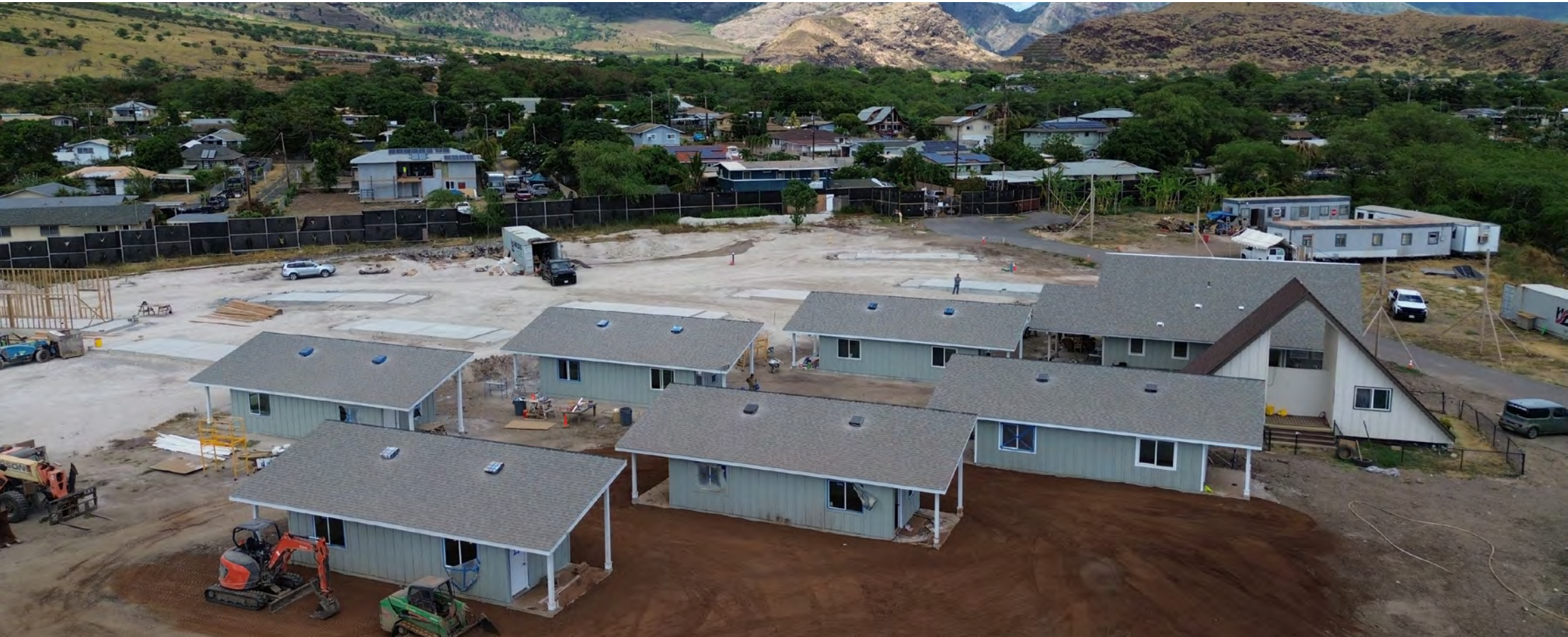
The Pu'uhonua O Wai'anae Farm Village is a mix of modernity and traditional Hawaiian communal living. So far, eight hale (homes) have been built this year with help and support from community partners. Pu'uhonua O Wai'anae hopes to support up to 250 people with a place to live when complete.
