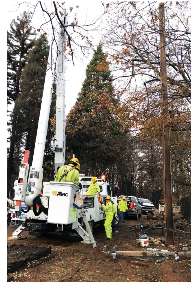
ABOVE: Crews from the Hawaiian Electric Companies frame poles in Northern California following the deadly Camp Fire.
