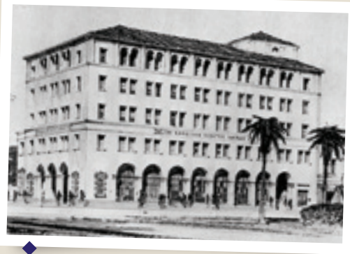
1927 Hawaiian Electric's King Street building opened for business on July 25.
