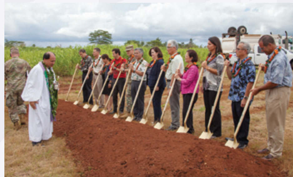
▲ Hawaiian Electric and the U.S. Army broke ground on a new power plant at Schofield Barracks that will strengthen the island's power grid and improve integration of renewable energy.
