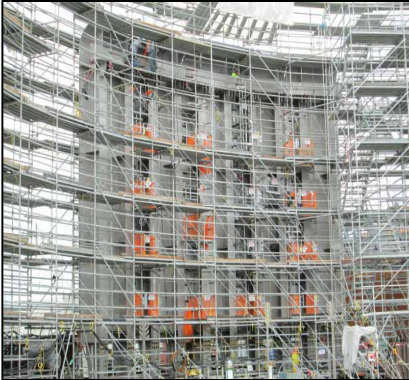
Unit 3 – CA03 module construction
