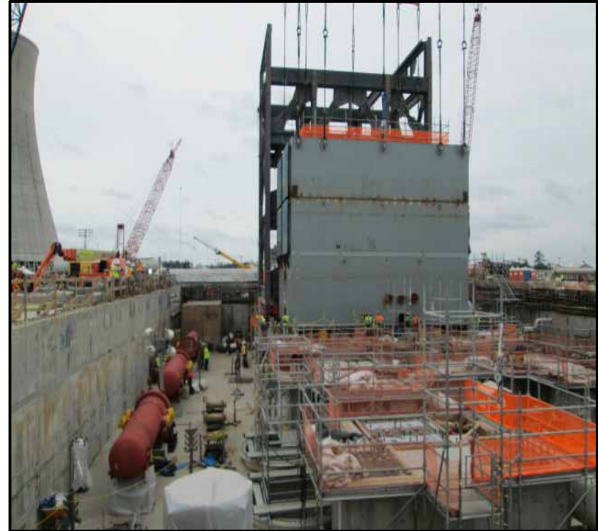
Unit 4 – Condenser installation
