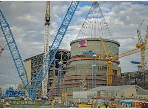
Unit 3 Final Containment Vessel Ring Set
