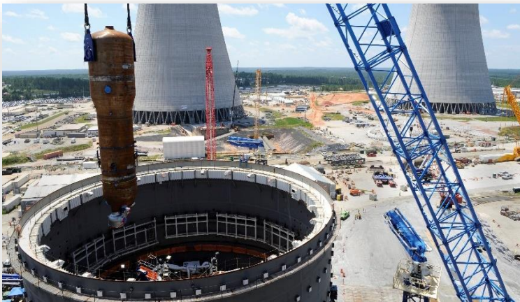
First steam generator placed inside Unit 3 containment vessel
