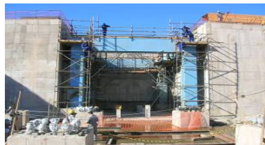
Apron feeder for primary crusher
