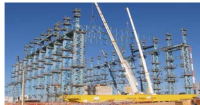
Erection of the grinding building
