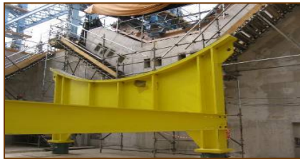
SAG mill cradle and foundation: August
