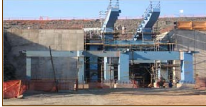
Primary crusher with structural steel installation in progress: September
