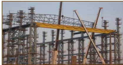
Grinding building structural steel: September
