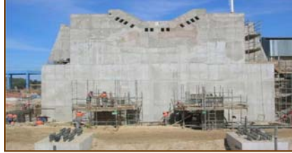
SAG mill foundation: June
