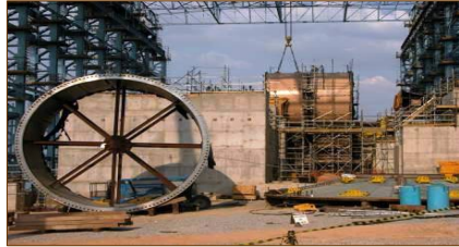
Ball mill progress: November 2007
