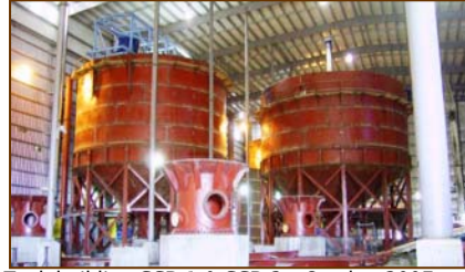
Tank building CCD 1 & CCD 2 - October 2007
