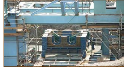
Crusher assembling in progress: October 2007
