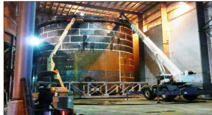
Leach tank fabrication – December 2007
