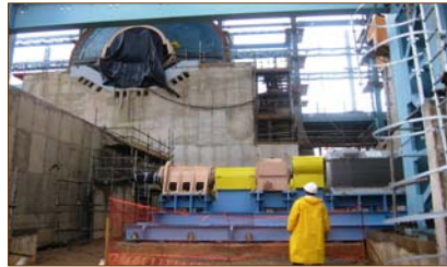
SAG mill progress: December 2007
