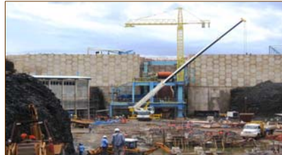
General view: December 2007
