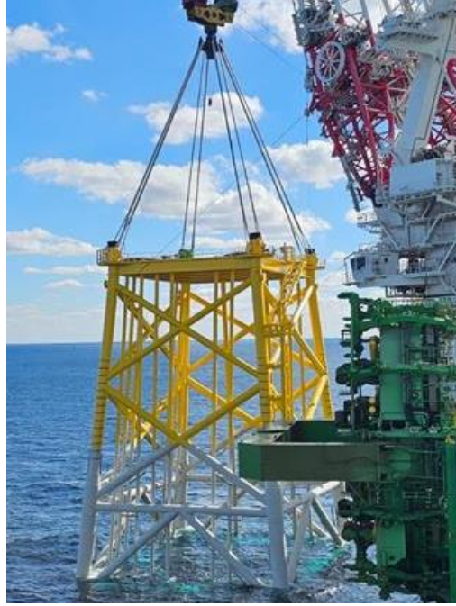
Second offshore substation jacket installation (October 2025)
