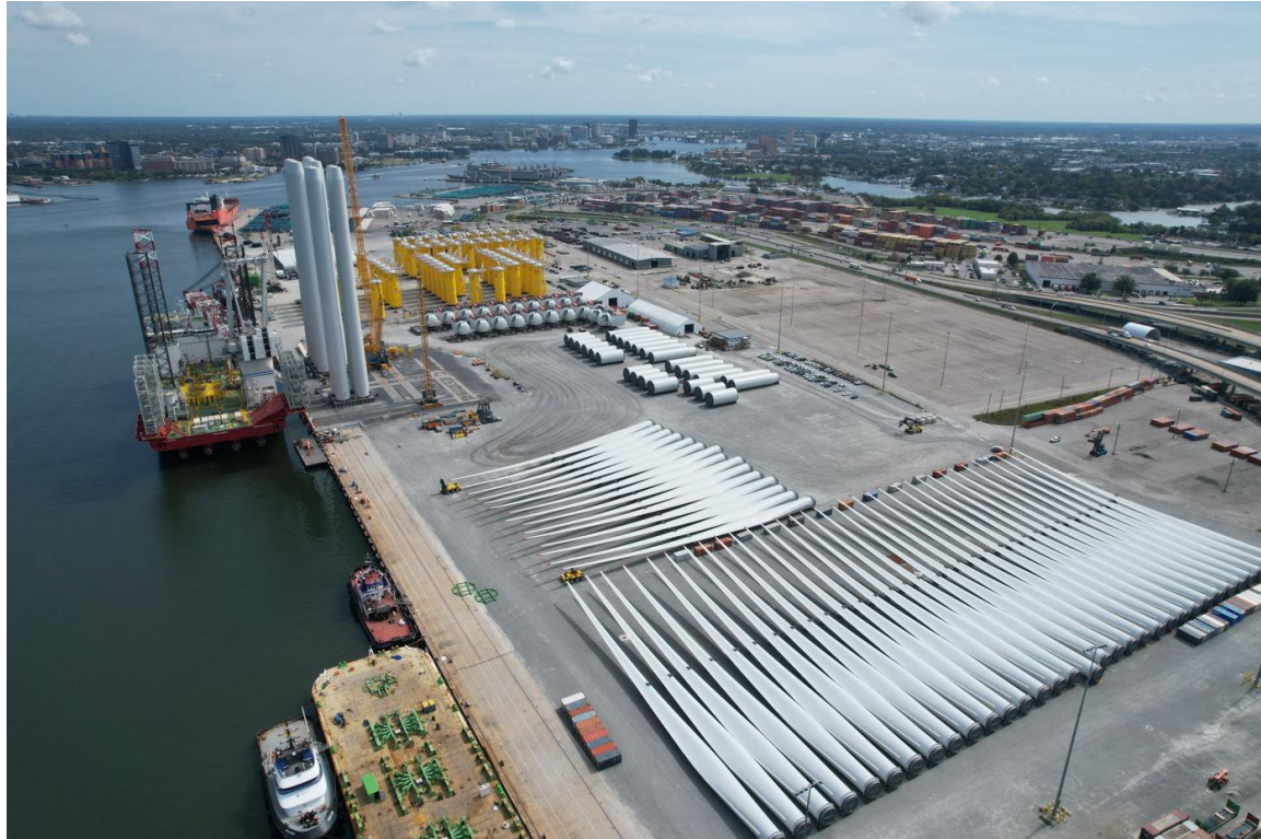
Component staging at Portsmouth Marine Terminal (October 2025)
