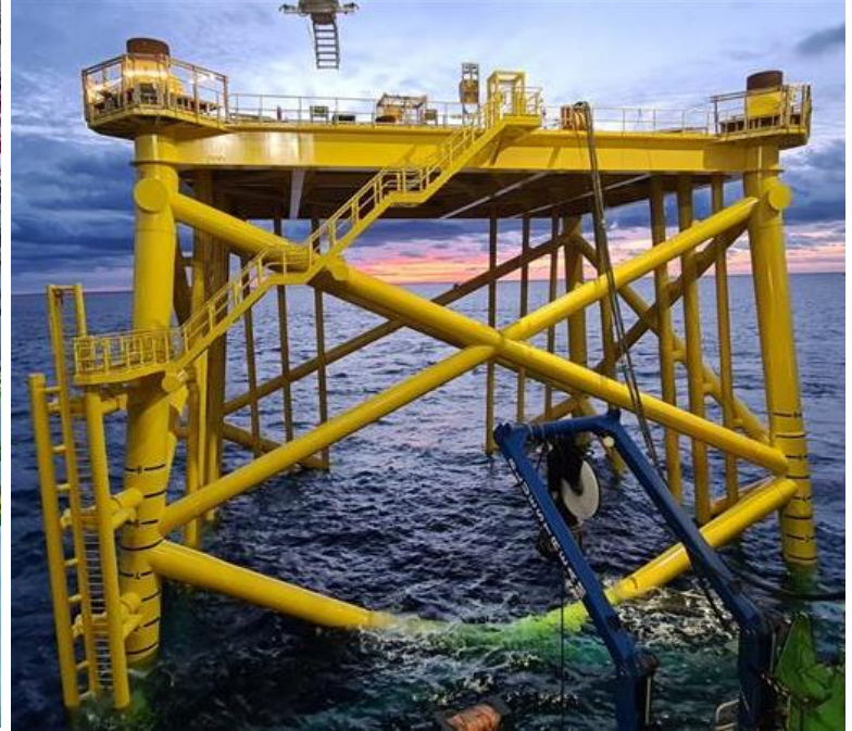
Second offshore substation jacket installation (October 2025)
