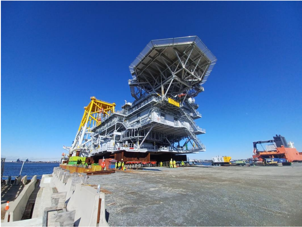
Third offshore substation at PMT (January 2026)
