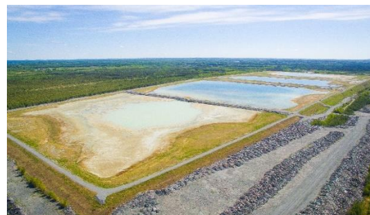
Rock Buttreassing at the Sigma Tailings Storage Facility, Canada
