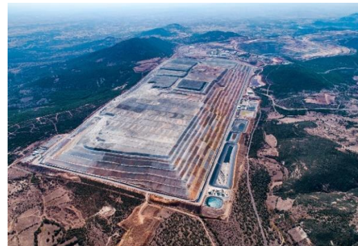
The Kışladağ Leach Pad, Turkey
