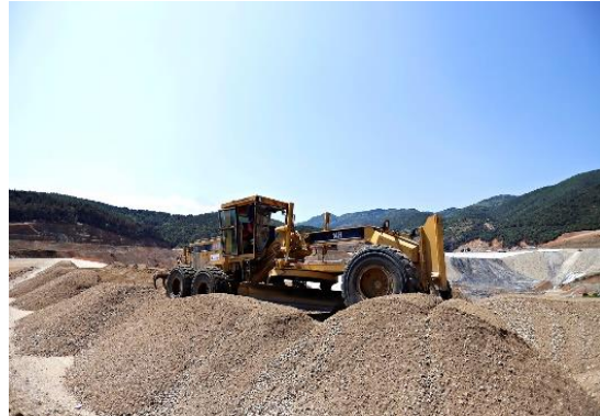
Dry-stack tailings at the Kokkinolakkas Tailings Management Facility, Greece
