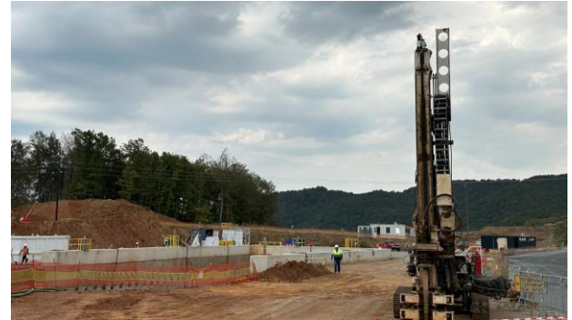
Primary crusher foundation
