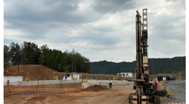
Primary crusher foundation
