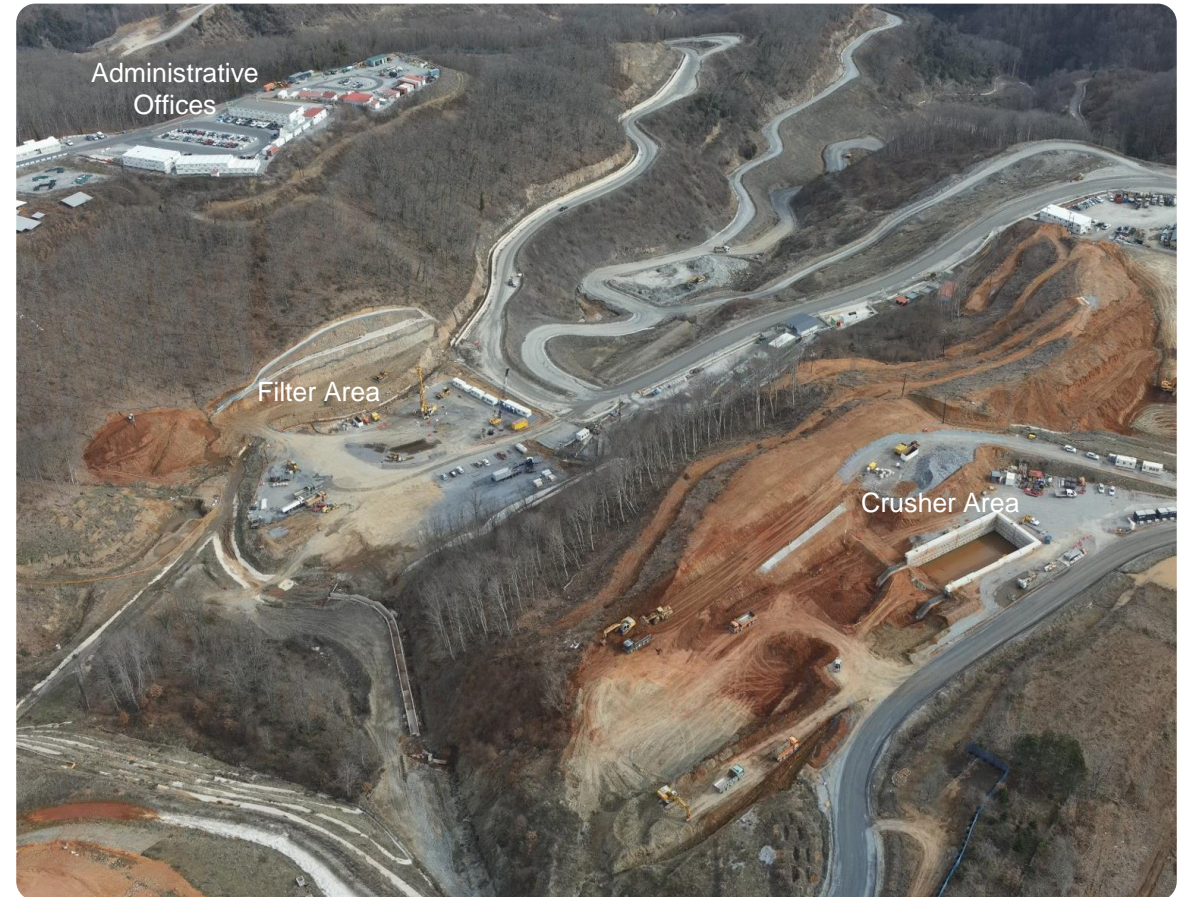
Aerial view of Skouries: January 2024
