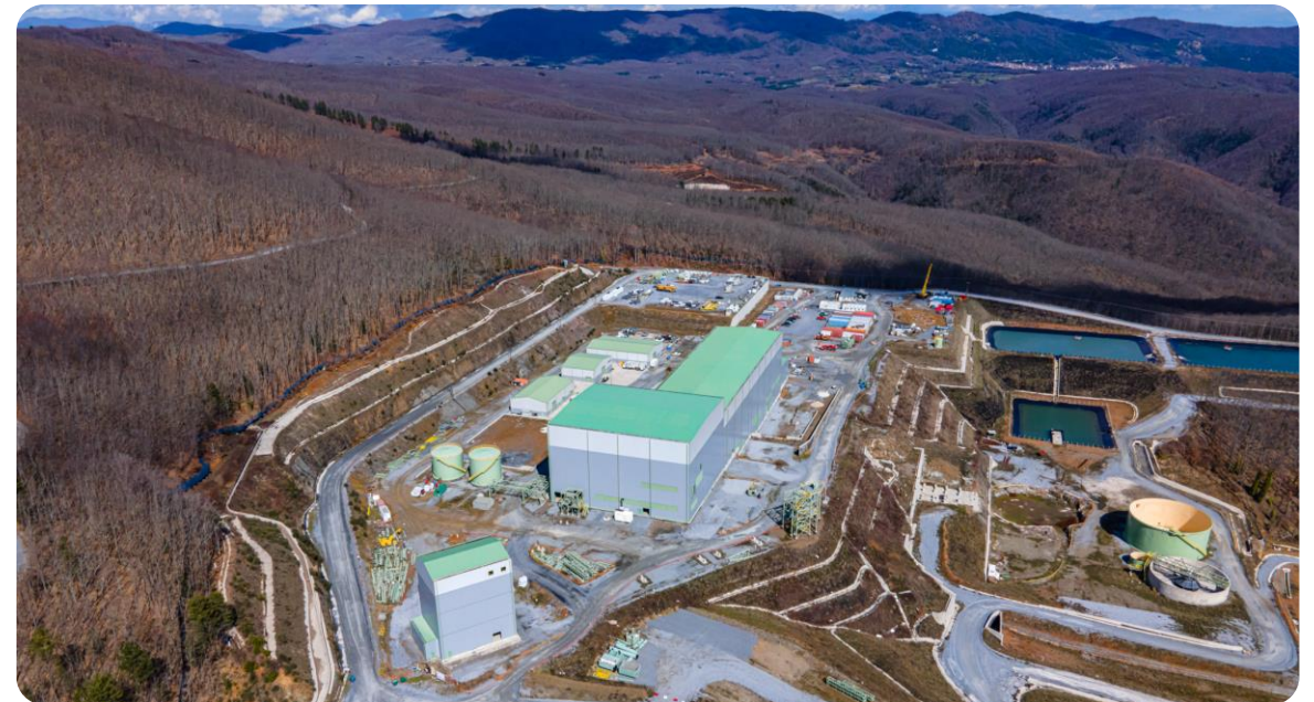
Aerial view of the mill building at Skouries.
