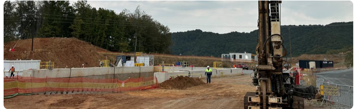
Primary crusher foundation
