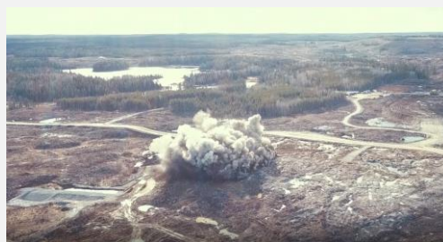
Initial open pit blast (May 2021)
