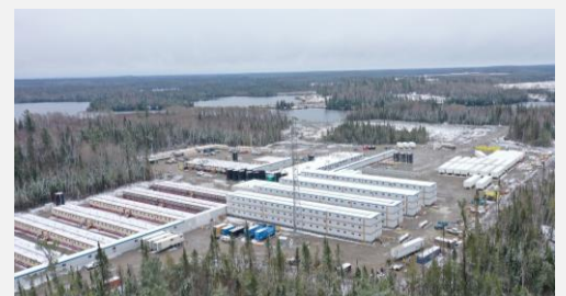
Permanent camp construction (May 2021)
