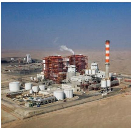
**3. Ocean cooling.** The desert location of the Angamos plant did not allow using potable water for the cooling tower. Instead, a seawater cooling tower was used, which runs at about two cycles of concentration. *Courtesy: AES Corp.*
